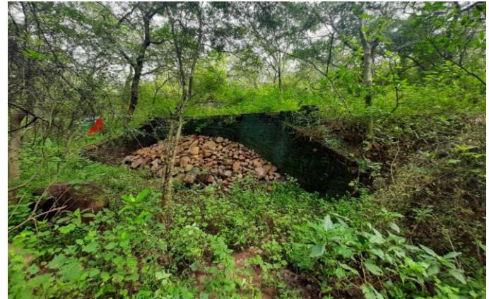
Bridge repurposed as check dam by Forest Department
